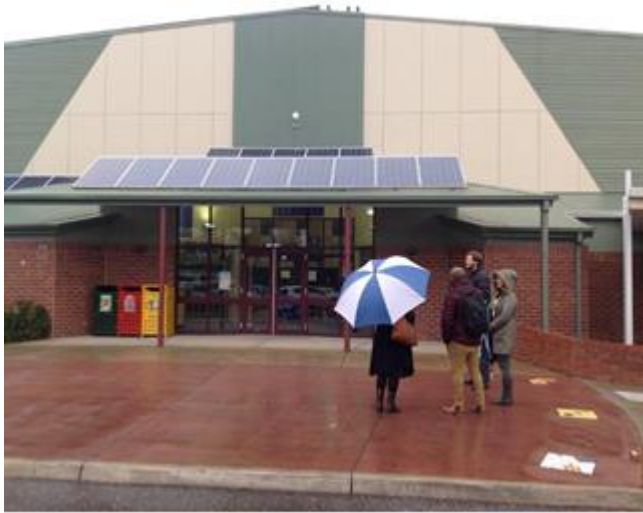
Figure showing solar-panels feeding back into electricity grid at school
