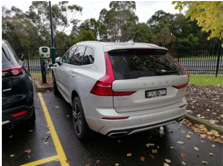
Figure showing Electric car charger station within the school premises
